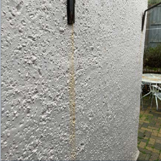
Metal archway causing paint discolouration.
